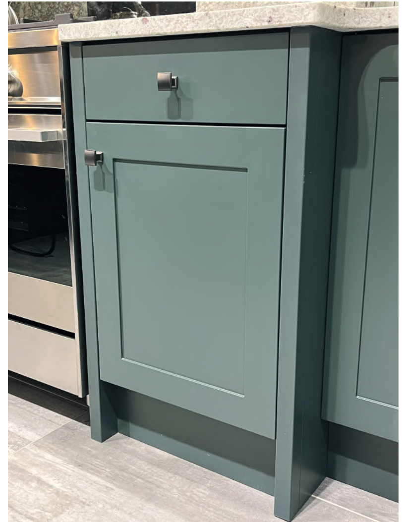
Variation in colour between the doors and the Universal Moulding.
