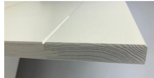
✓ DOOR EDGE - END GRAIN PAINT COVERAGE
